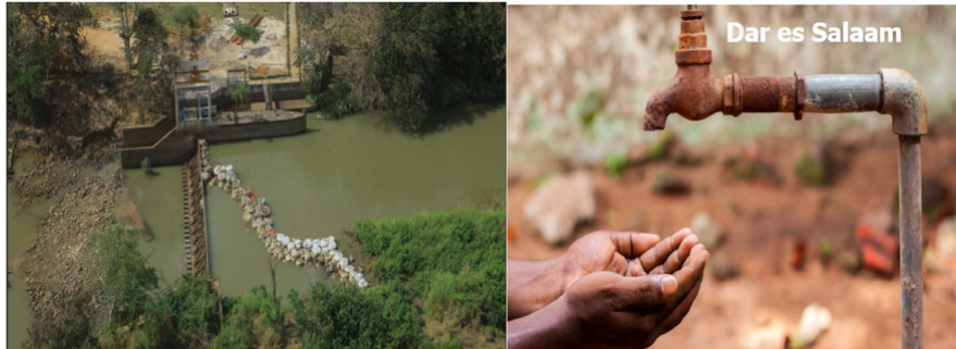
Impact of the 2021/22 Critical Hydrological Drought at the Lower Ruvu DAWASA Treatment Plant.
