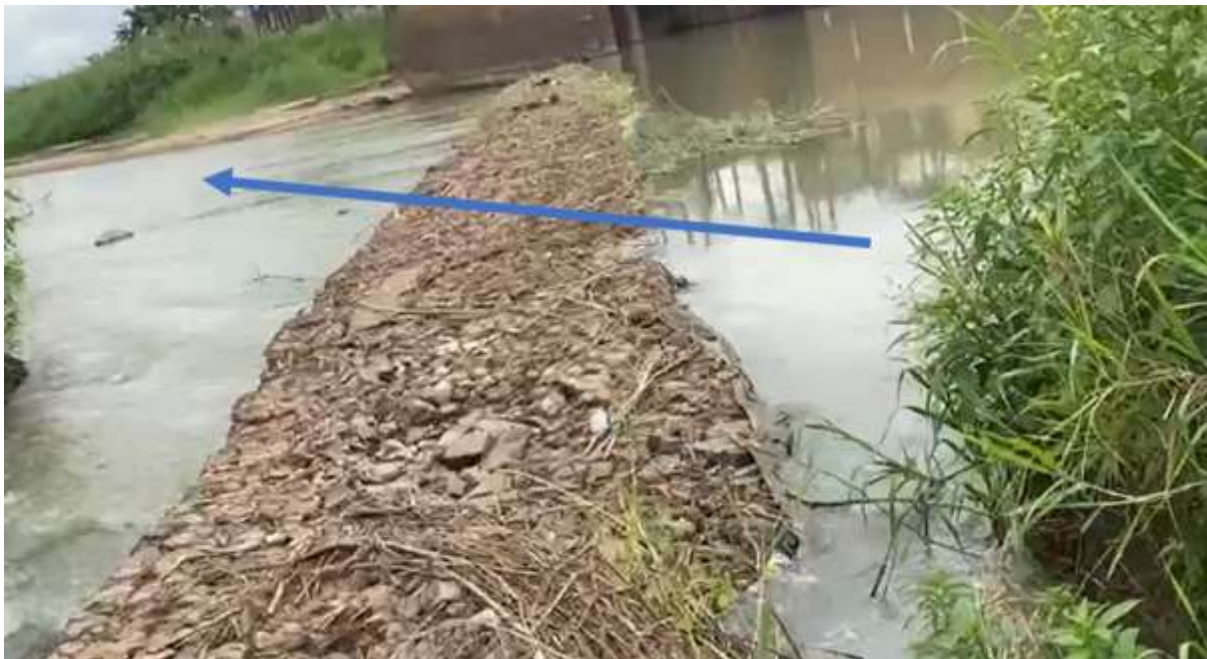
The water diversion weir constructed in year 2022 downstream of the 1H&A flow gauging station, which rendered the existing rating curve useless.
